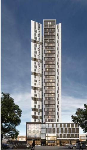
EXISTING MIXED USE DEVELOPMENT "Meriton Suites" 33 storey mixed use development 163 service apartments & child care
