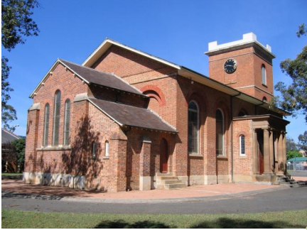
ST LUKE'S ANGLICAN CHURCH Heritage-listed Anglican church built in 1820
